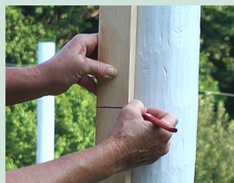
STEP 1 Mark posts with desired placement.
