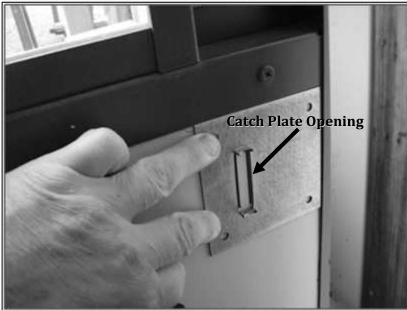
Drill out the traced slot and attach the catch plate to the door. Be careful not to drill too far and damage the other side of the door. A 1 1/4" hole bit works well.
