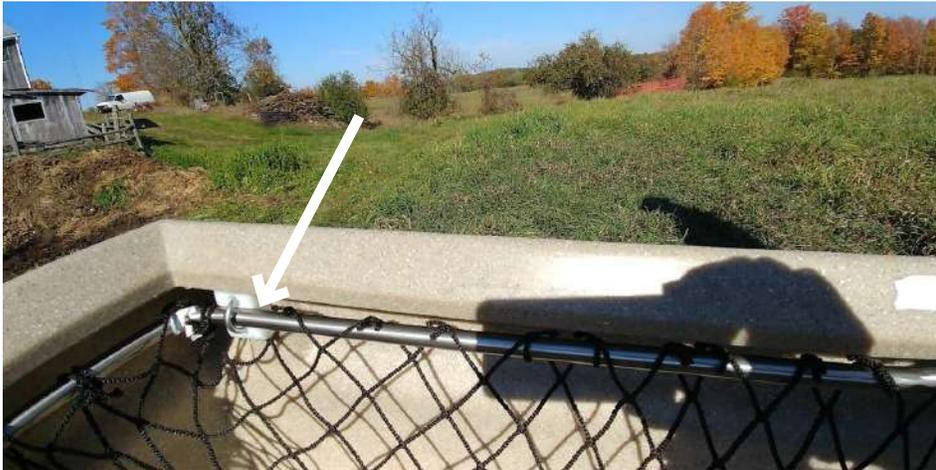
4. Remove the 4 nuts & washers on the U-bolts using the 7/16" socket or wrench.
