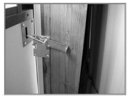
Attach Jamb Latch to the jamb and adjust as needed.
