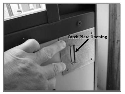
Drill out the traced slot and attach the catch plate to the door. Be careful not to drill too far and damage the other side of the door. A  $1 \frac{1}{4}$  hole bit works well.
