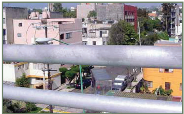
Gray coating due to processing (Acceptable)
