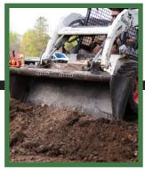
Expand panels to relax for installation. Prepare & compact subgrade to repair pre-existing ruts & support drainage.
