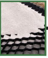
Infill Mud Management cells with crushed gravel.
