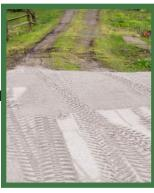
Overfill, water, & compact area with topsoil or stone of your choice.
