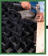
Connect & secure panels with stakes. Secure & protect your edges with a structural border. (example: pressure treated lumber)
