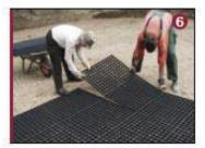
Start laying down the grids with the tabs facing the direction of laying process. The grids self-lock by snapping in with the attached tabs.
